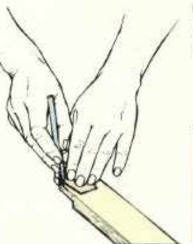
1 Mark the dovetail slope
